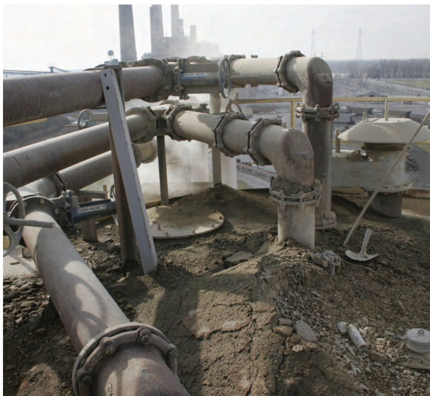
Roof of silo at fly-ash processing plant
