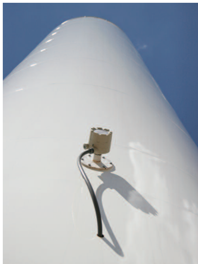
Rotary paddle level sensor installed on vessel wall
