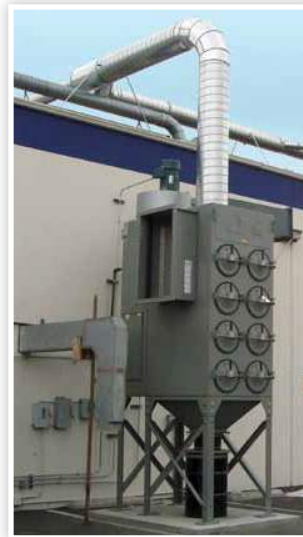
DustHog SFC 16-4 used for blending nutritional powders.
