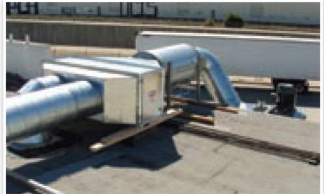
Exhaust duct from the DustHog SFC downward flow dust collector with in-line silencer and safety filter.
