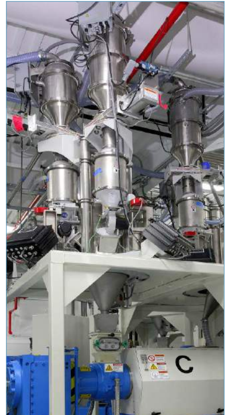
Loss-in-weight blending system with vacuum receivers mounted above a weigh-hopper on a single screw extruder, the third extruder on five-layer coextrusion sheet line ruder., the third extruder in a five-layer coextrusion sheet line.
